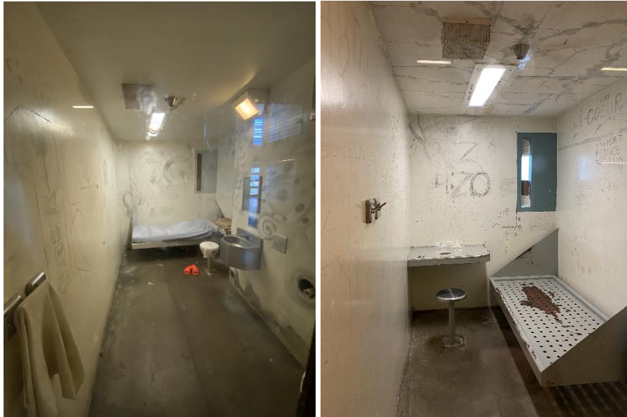
Photographs 4 and 5: Administrative Segregation / Disciplinary Isolation Cells
