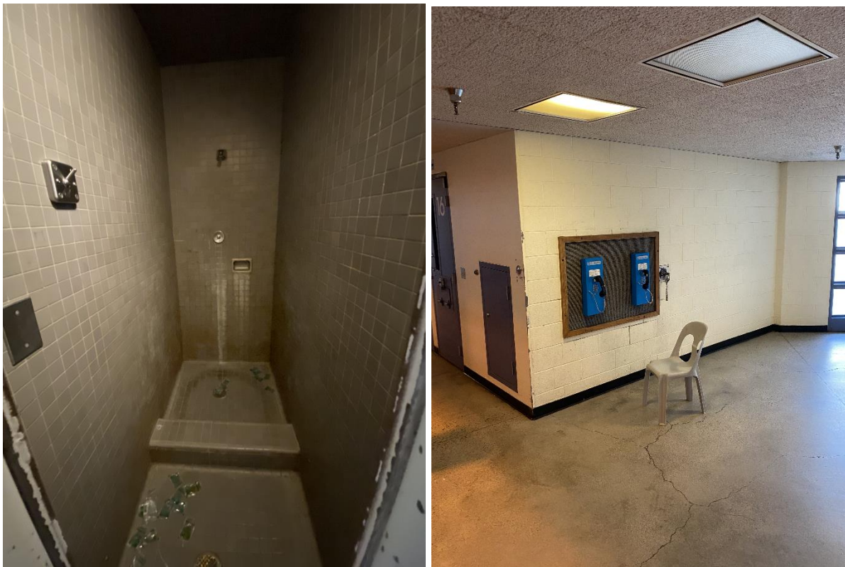
Photographs 8 and 9: Non-ADA Shower in AS7 with trash; Inaccessible Phones in Medical Housing
