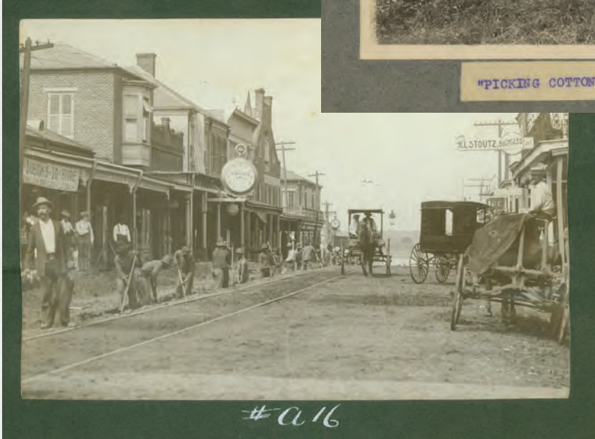
Men digging a trench to install sewerage line on Main Street, circa 1900 (Andrew David Lytle Sr./State Library of Louisiana)
